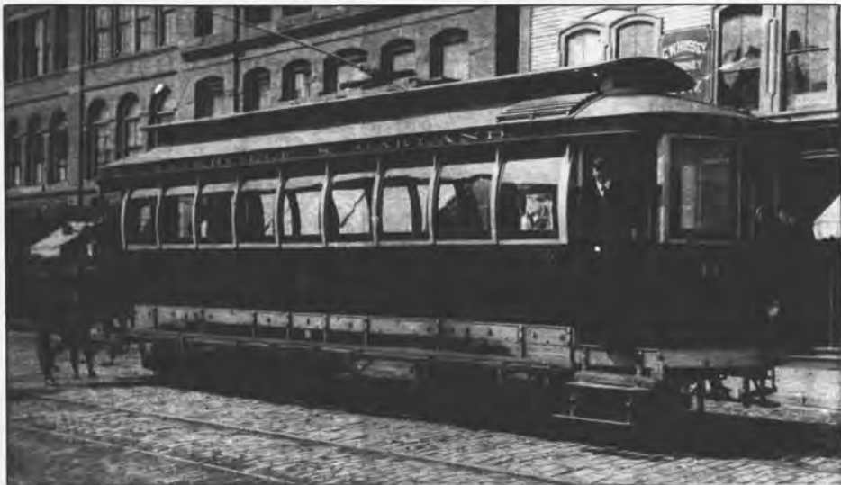
One of the electric trolleys, with its crew, Mel Beane and Joseph Jordan.
