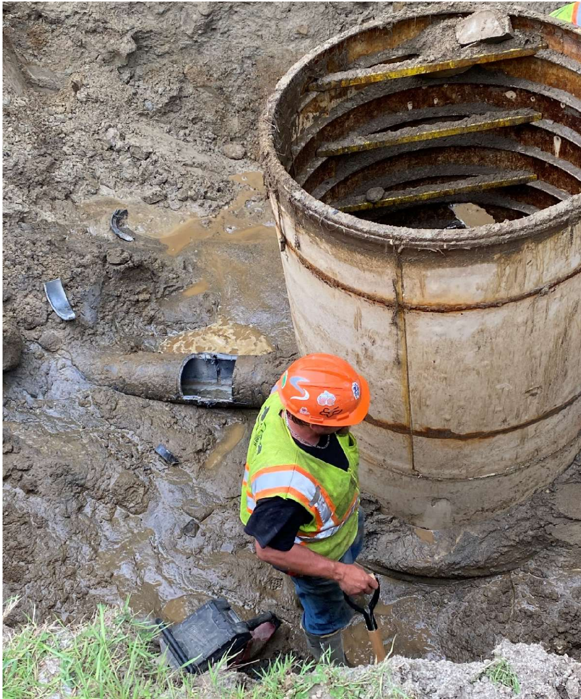
Figure 1- Sawtelle Road SMH Replacement May 23, 2024
